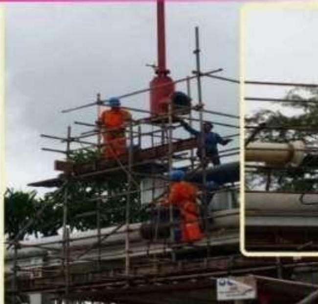
Preparation for Pipe Spool Temporary & Vlt up Ball Valve
